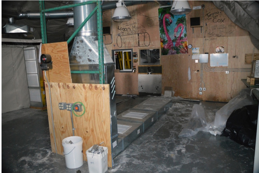
View of what's remaining inside of the core handling arch. Photo: Don Voigt.
