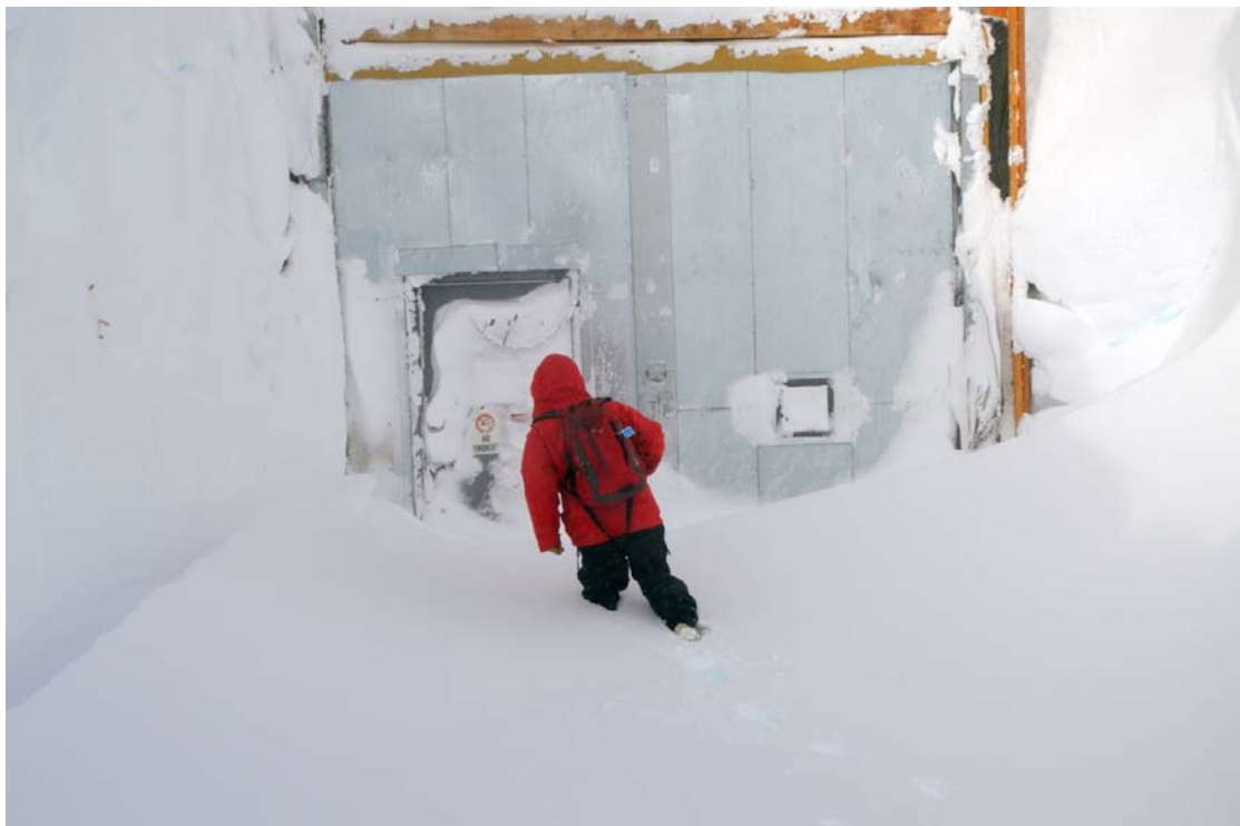
Heavy drifting at the doors to the drilling side of the arch. Photo: Don Voigt.
